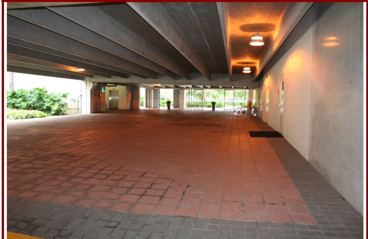
VIEW OF THE PARKING GARAGE INTERIOR
