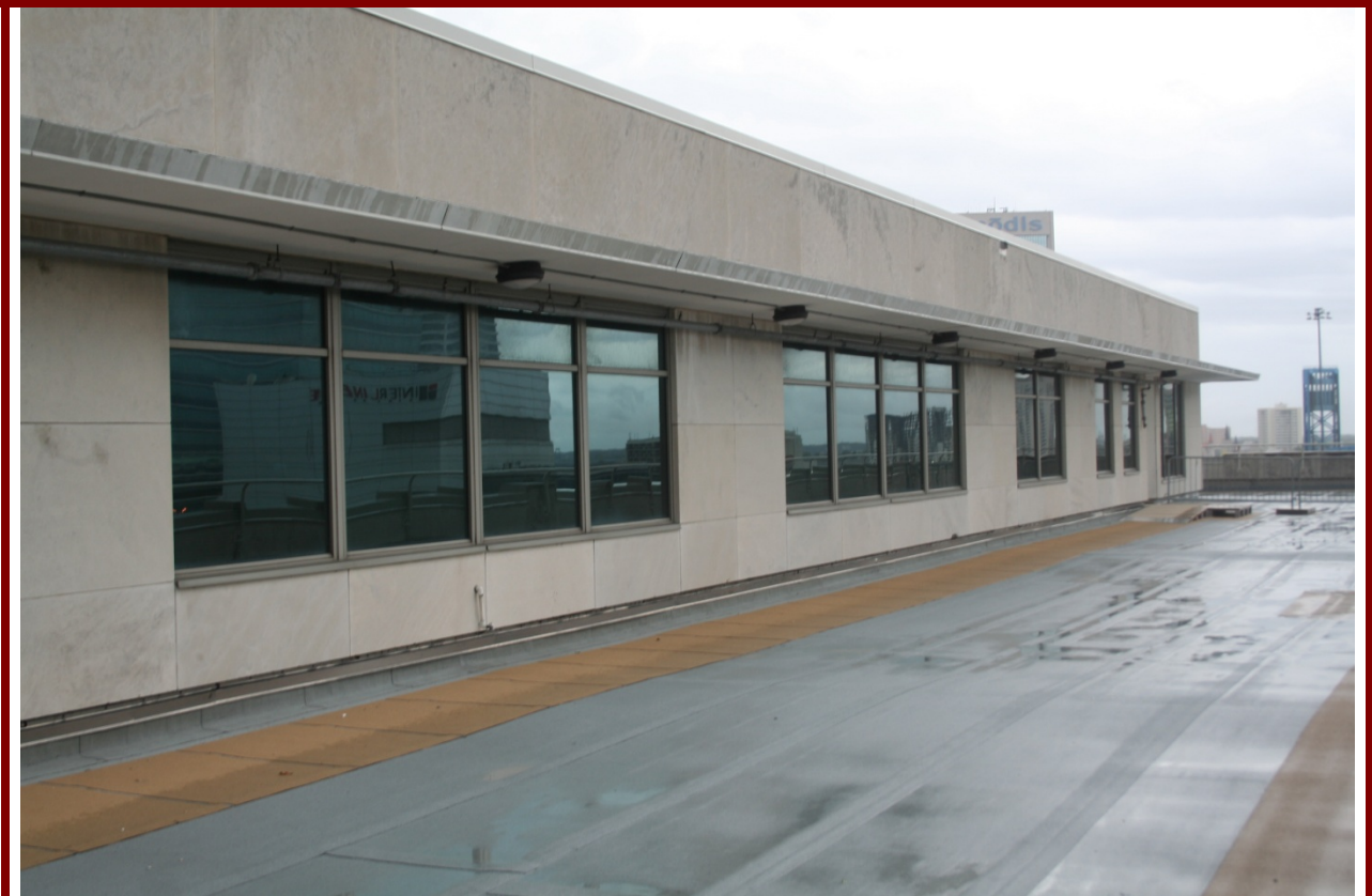
VIEW OF ROOF AREA
