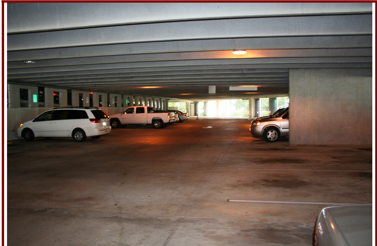
VIEW OF THE PARKING GARAGE INTERIOR
