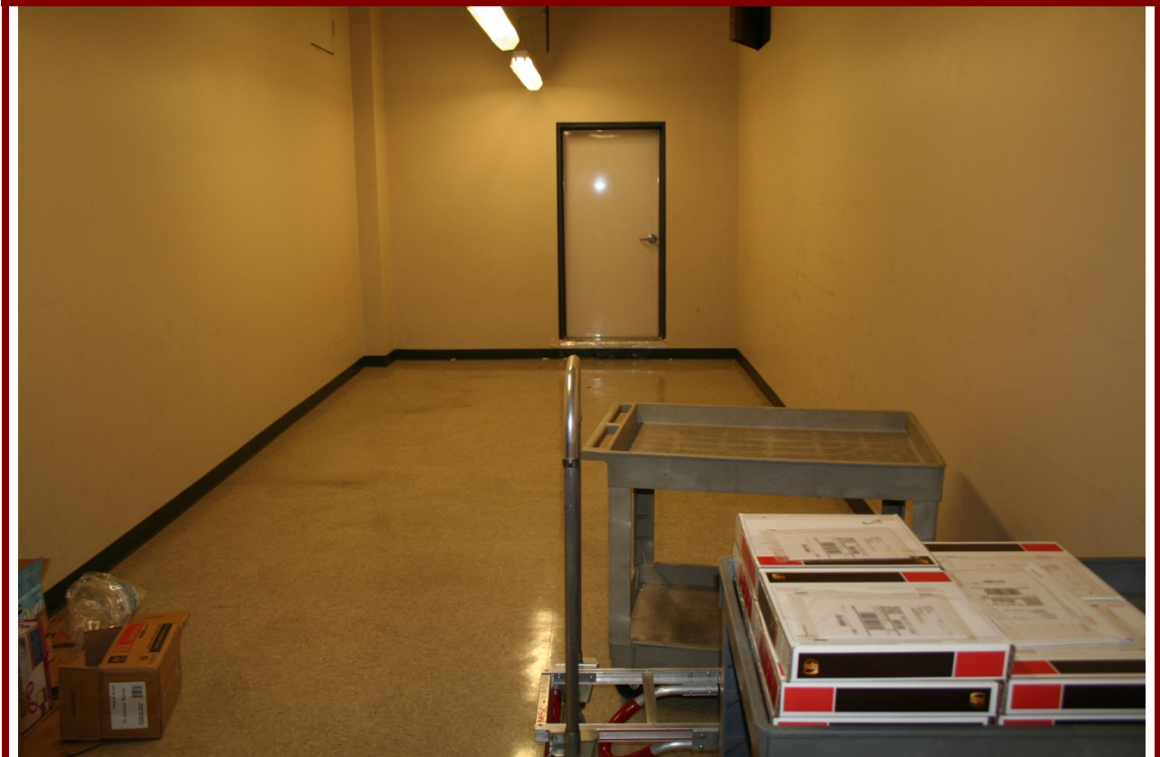
VIEW OF A TYPICAL SERVICE HALLWAY
