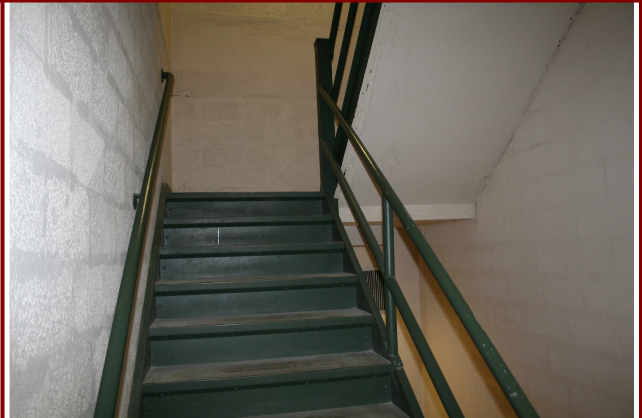
VIEW OF TYPICAL UNFINISHED STAIR CORE
