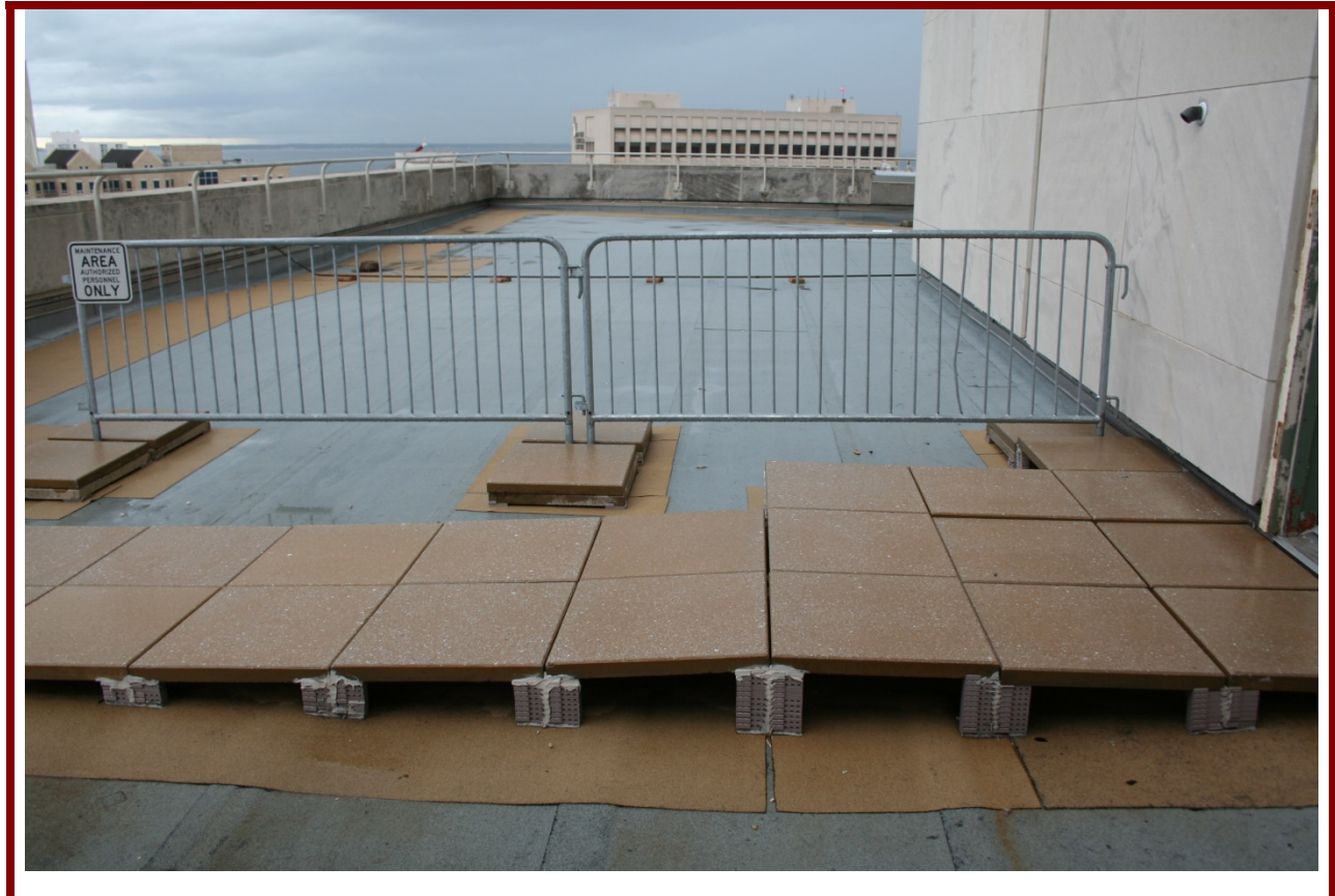
VIEW OF ROOF AREA
