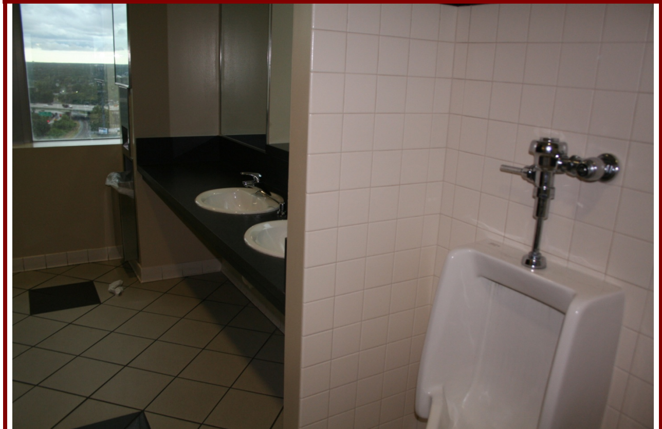
VIEW OF REPRESENTATIVE FINISHED REST ROOM AREAS
