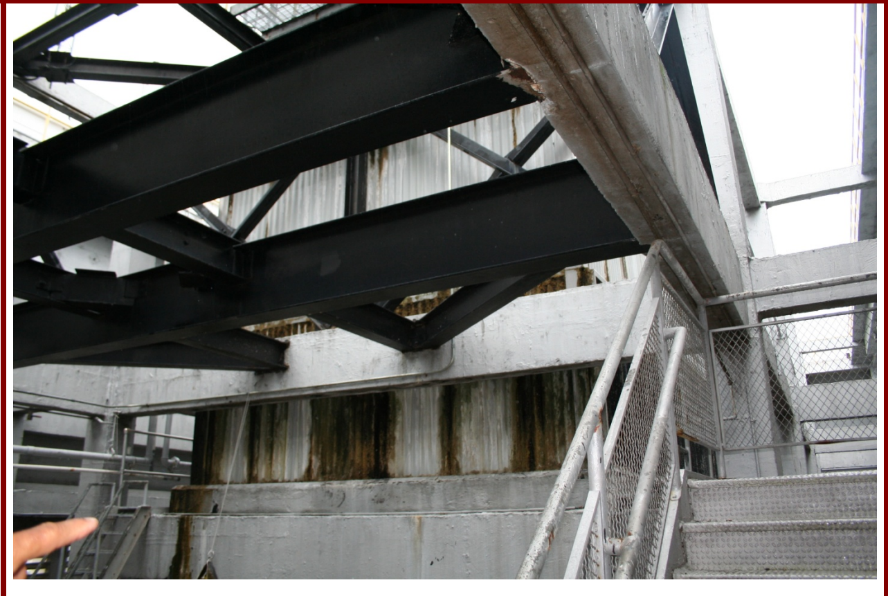
VIEW OF COOLING TOWER
