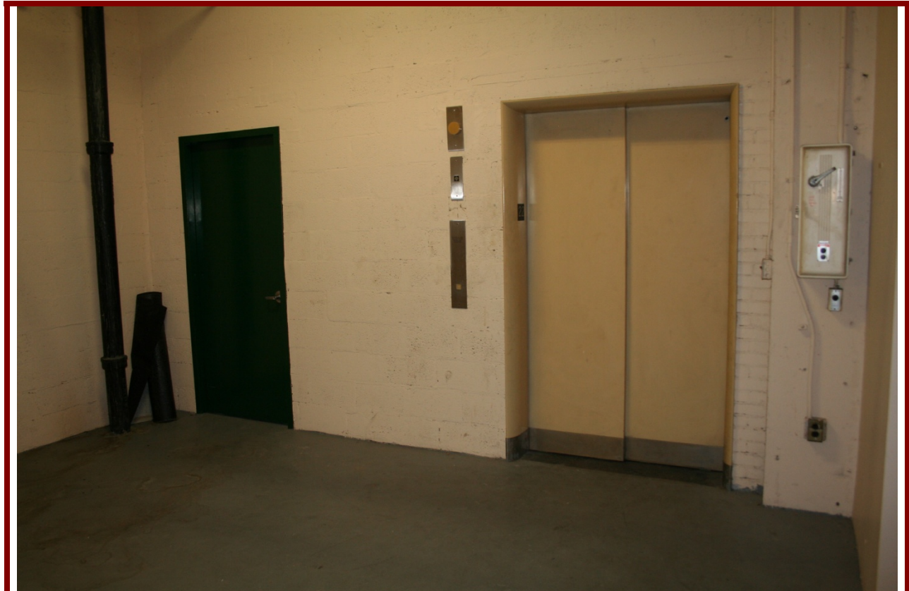
VIEW OF TYPICAL SERVICE ELEVATOR LOBBY
