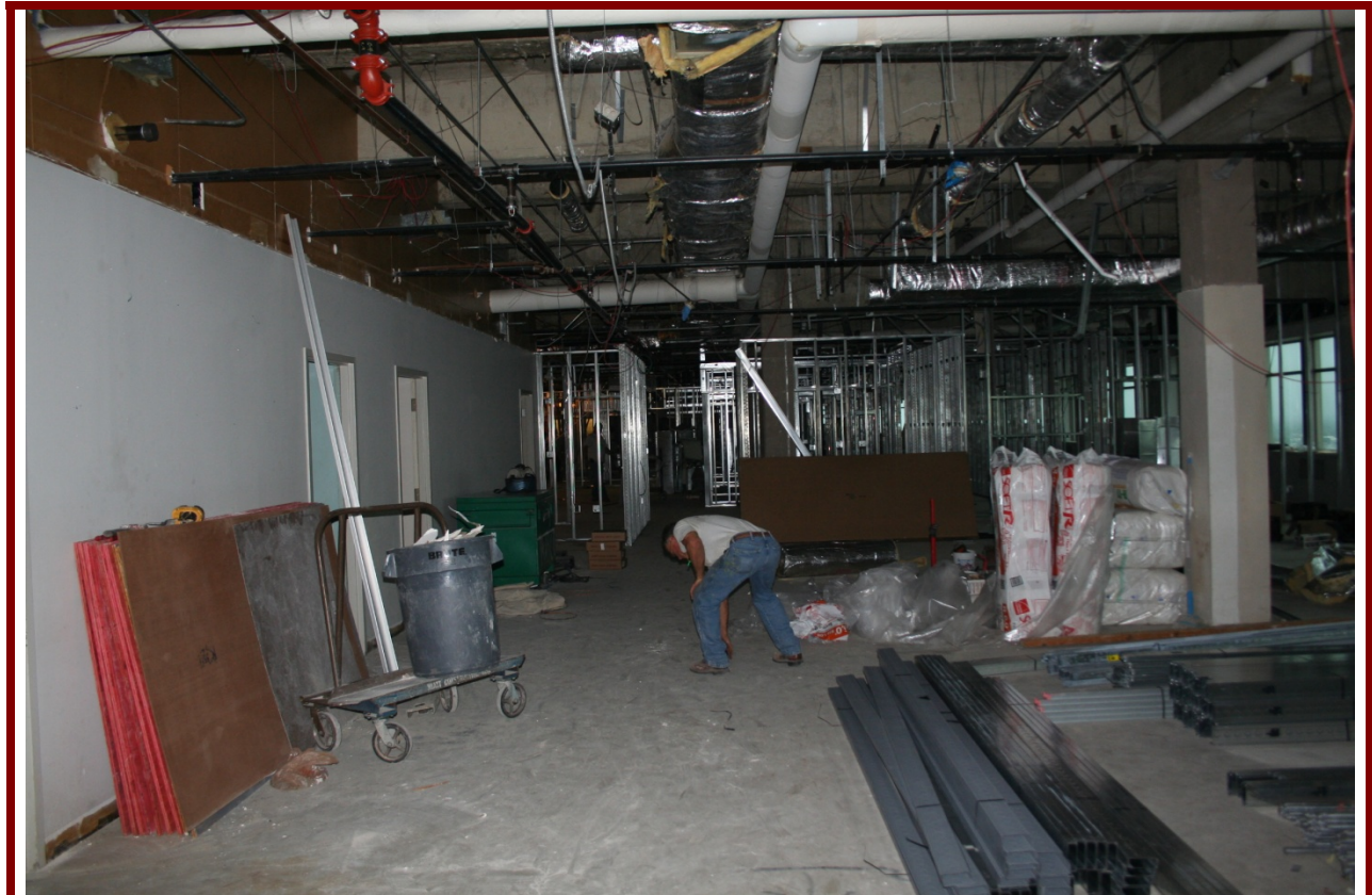
VIEW OF UNFINISHED TENANT SPACE UNDERGOING BUILDOUT
