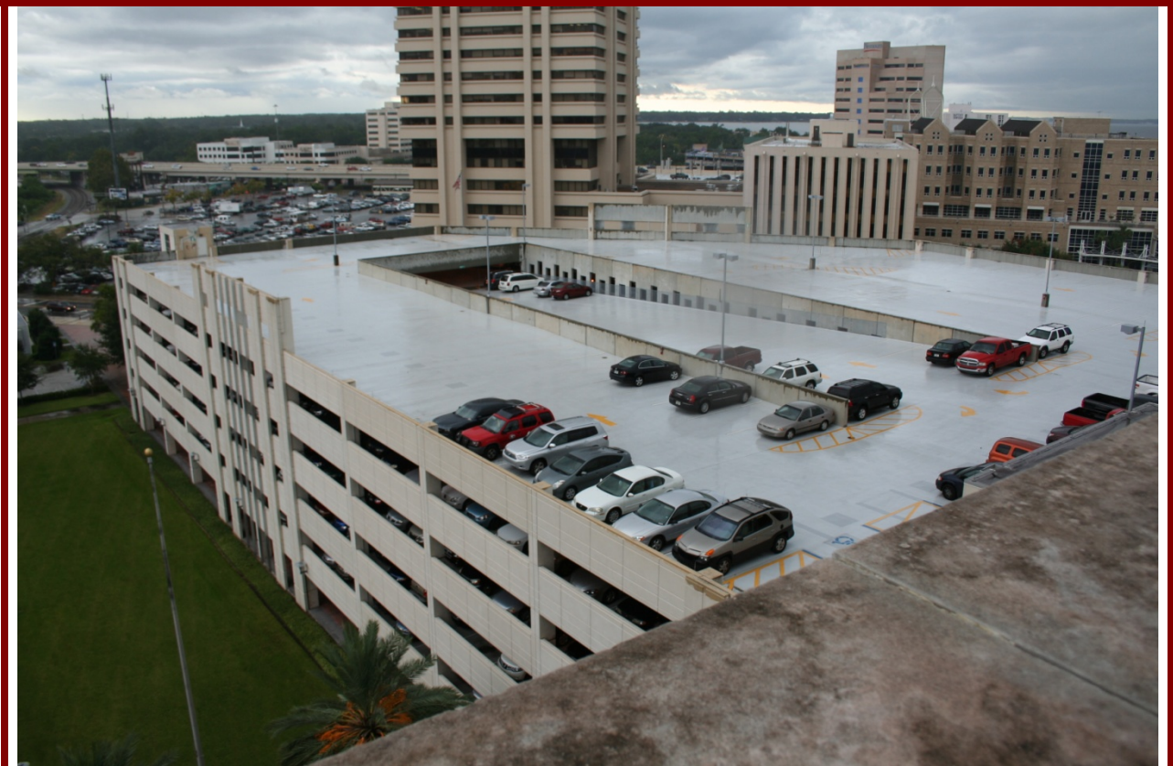
VIEW OF THE PARKING GARAGE UPPER DECK
