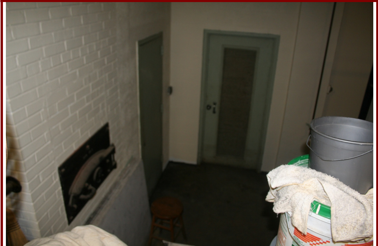
VIEW OF BASEMENT AREA
