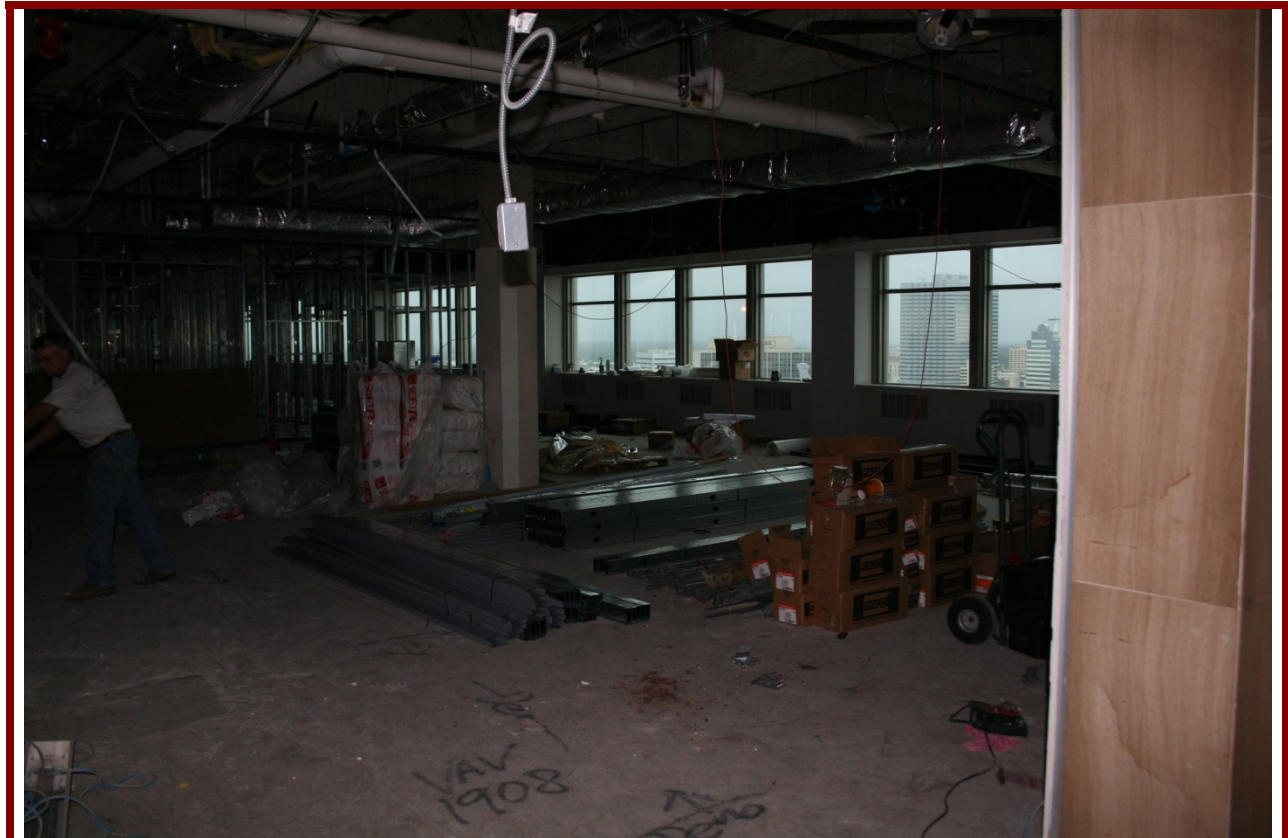
VIEW OF UNFINISHED TENANT SPACE UNDERGOING BUILDOUT
