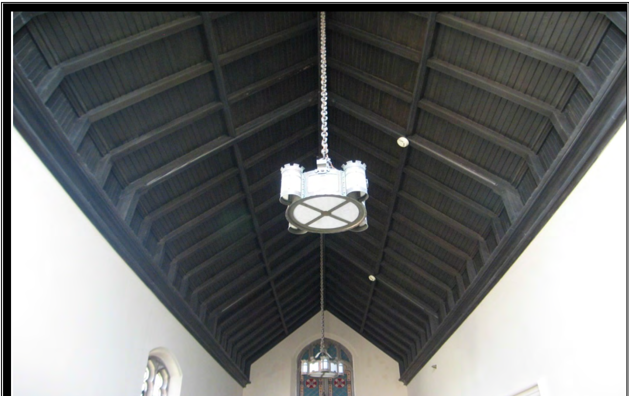
INTERIOR VIEW OF PARISH HALL BUILDING
