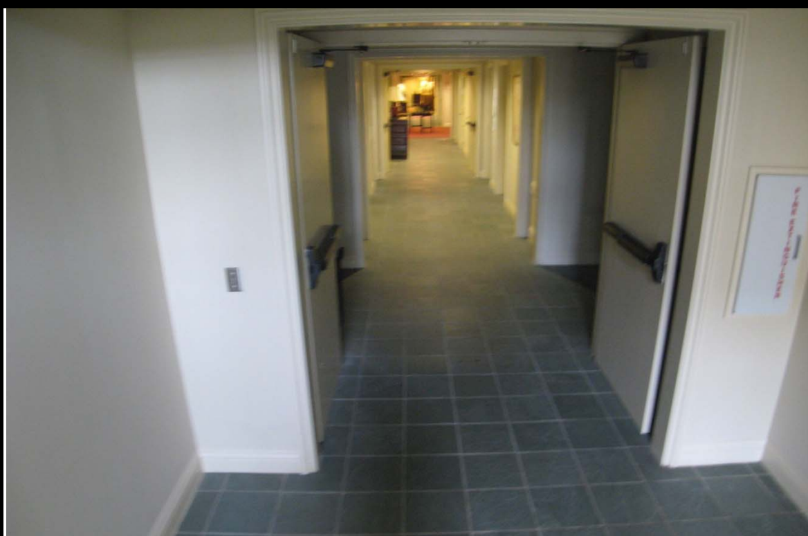
INTERIOR VIEW OF THE NEW EDUCATION BUILDING
