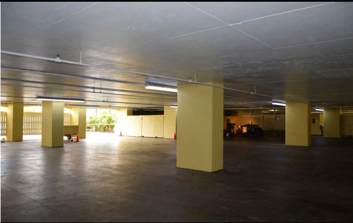
VIEW OF PARKING AREA AT BUILDING A #1
