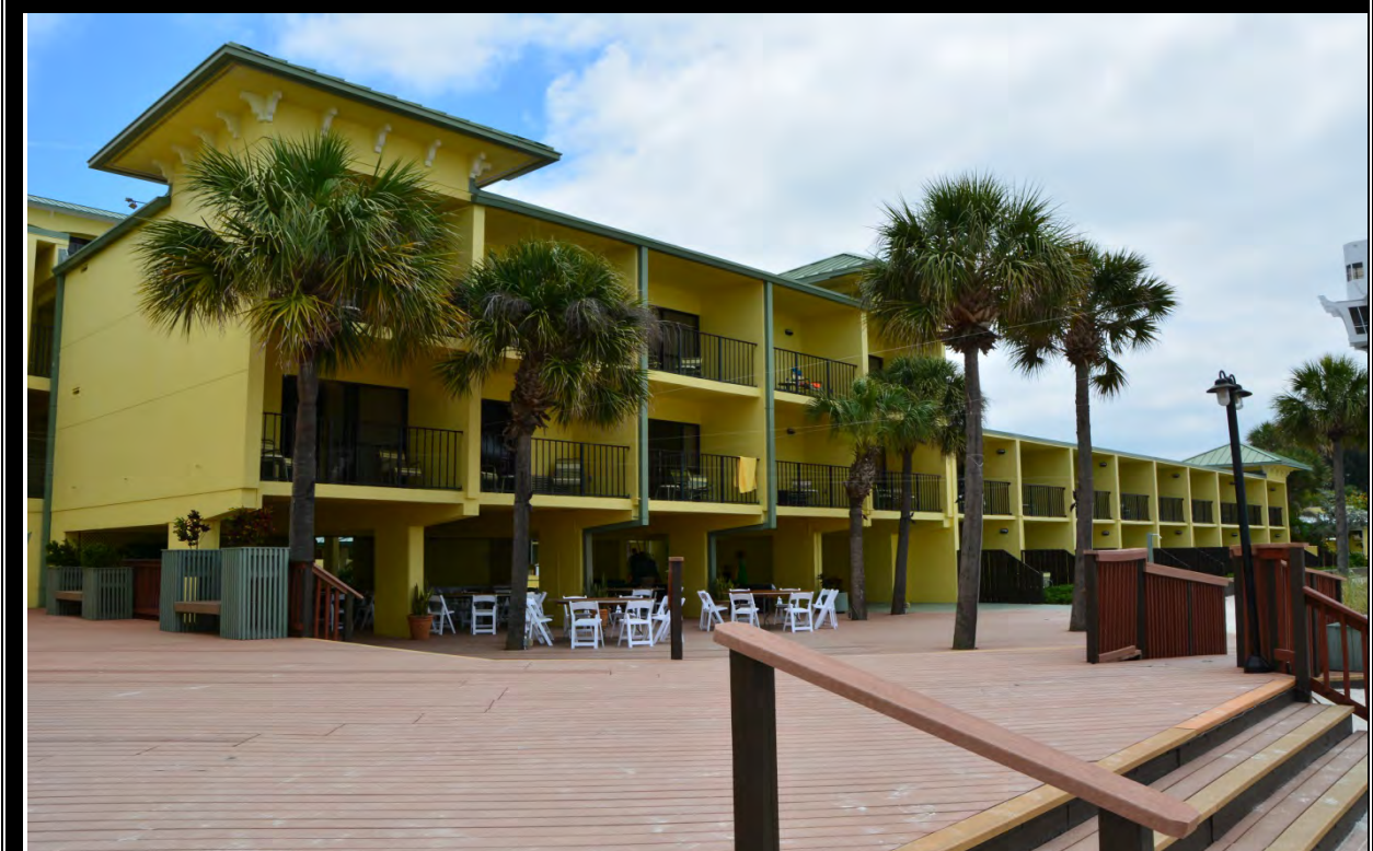
EXTERIOR VIEW OF BUILDING D #2 & E #2A
