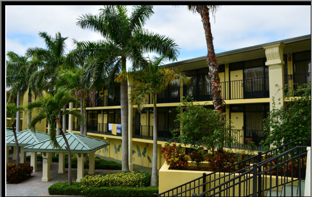
EXTERIOR VIEW OF BUILDING D #2 & E #2A
