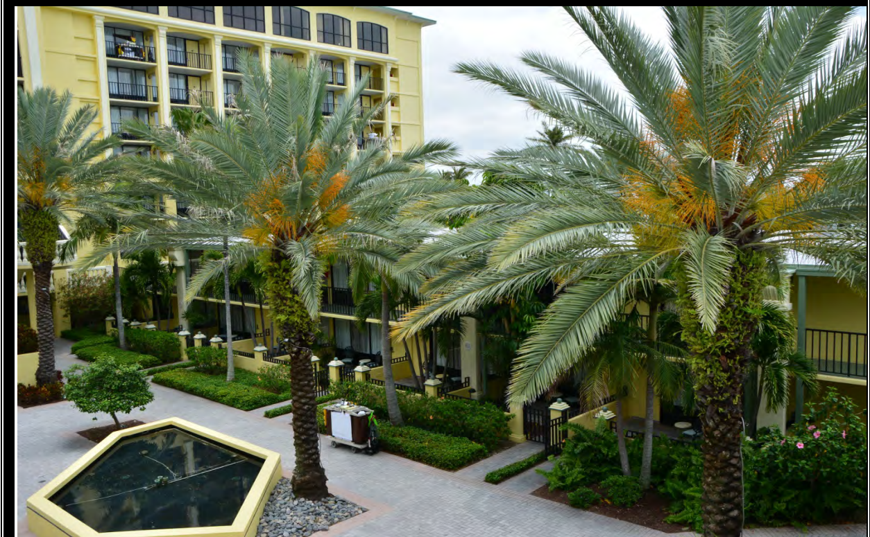
EXTERIOR VIEW OF BUILDING D #2 & E #2A
