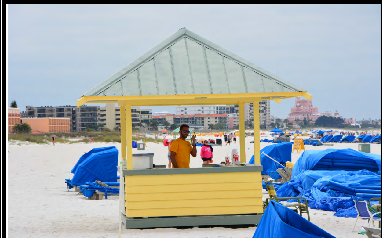
VIEW OF BEACH CABANA RENTAL STRUCTURE
