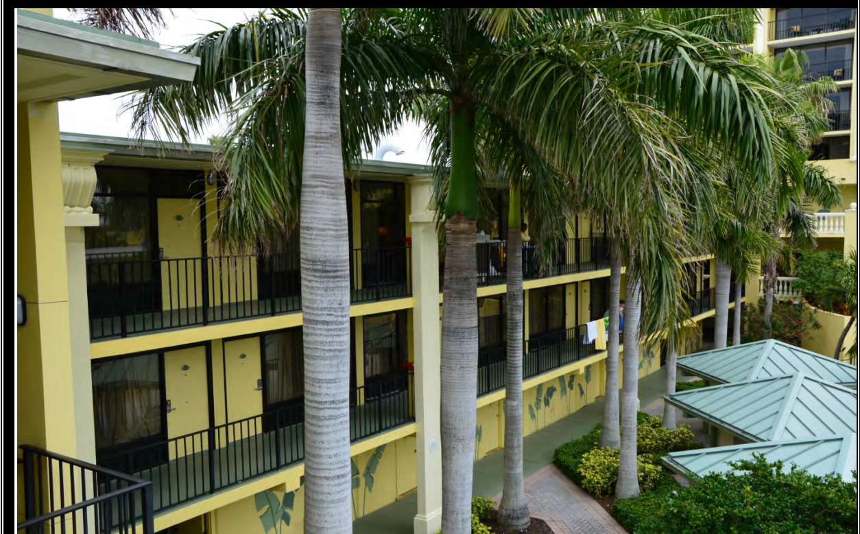
EXTERIOR VIEW OF BUILDING D #2 & E #2A
