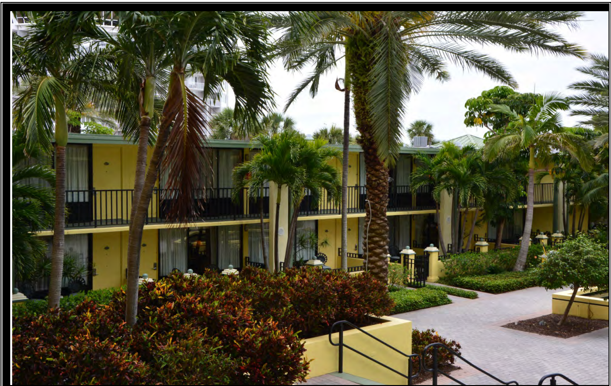
EXTERIOR VIEW OF BUILDING D #2 & E #2A
