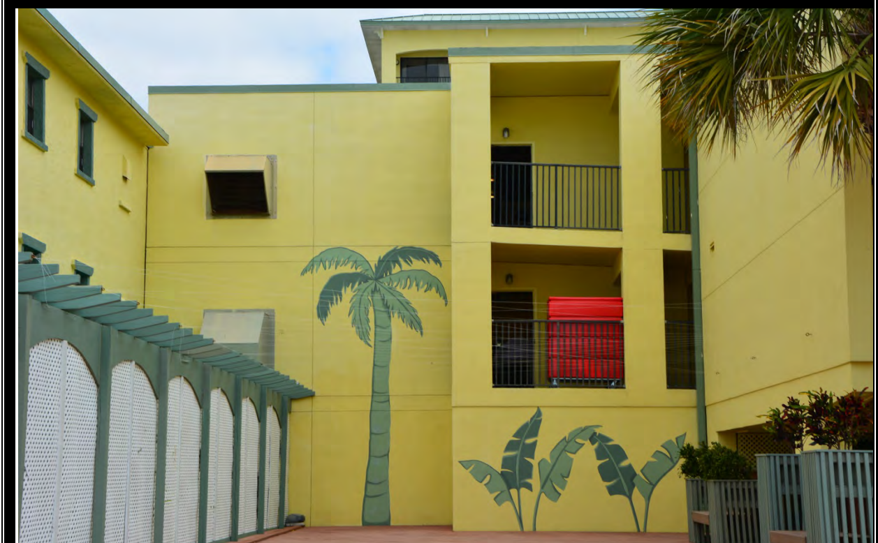
EXTERIOR VIEW OF BUILDING H/#2B – HOUSEKEEPING AND MAINTENANCE AREA
