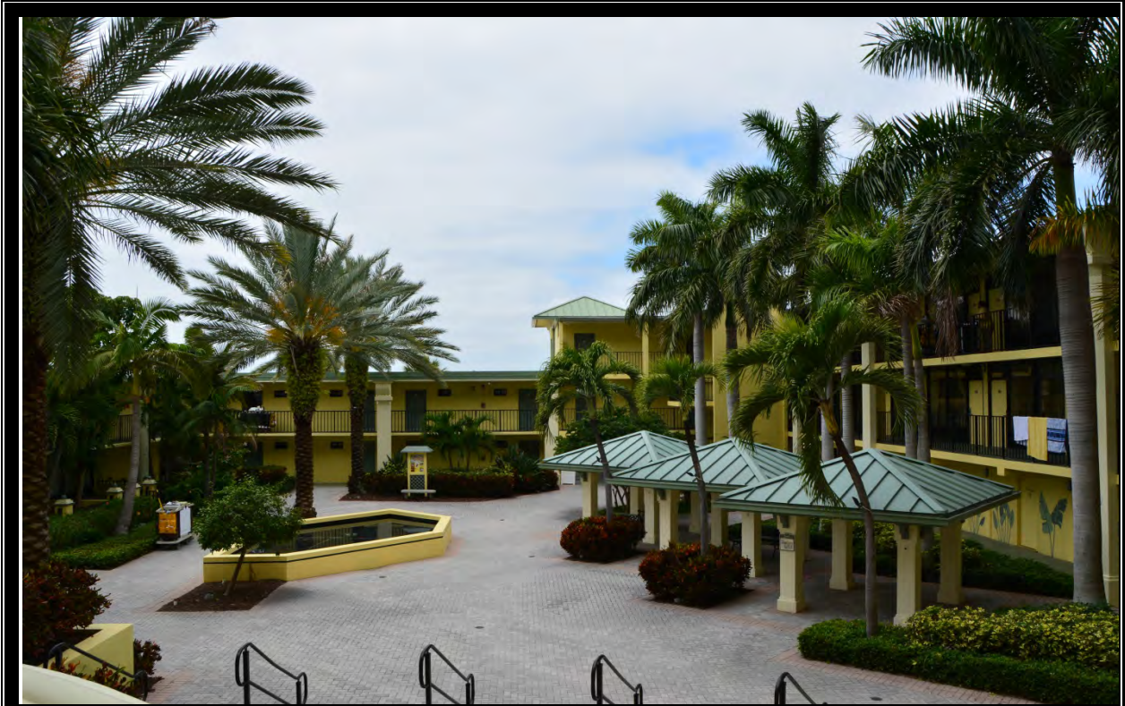
EXTERIOR VIEW OF BUILDING D #2 & E #2A
