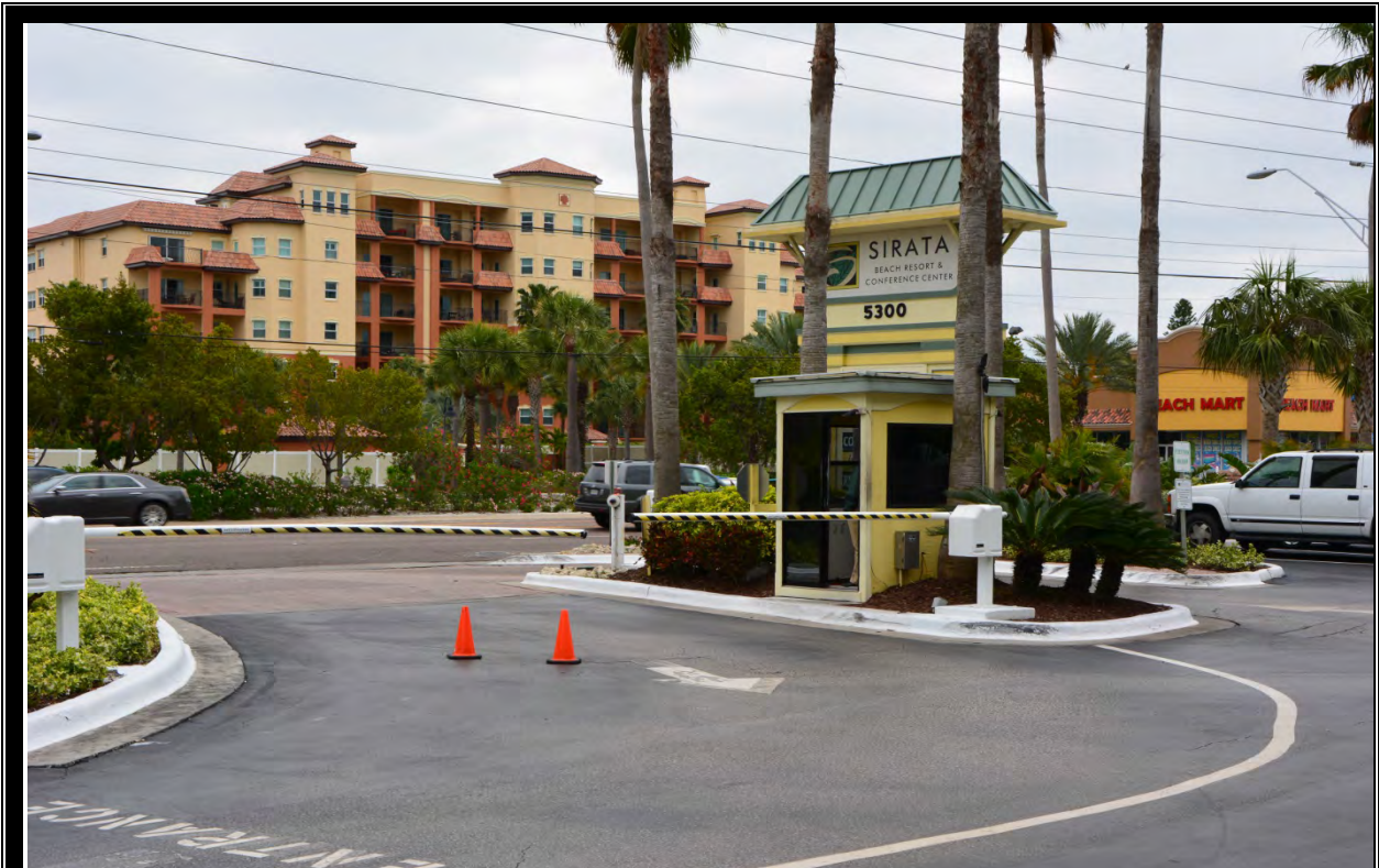
VIEW OF GUARD HOUSE AND ENTRY/EXIT SYSTEM
