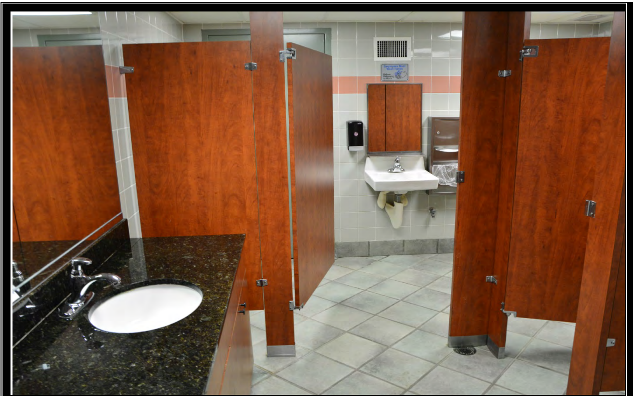
VIEW OF TYPICAL COMMON AREA RESTROOM
