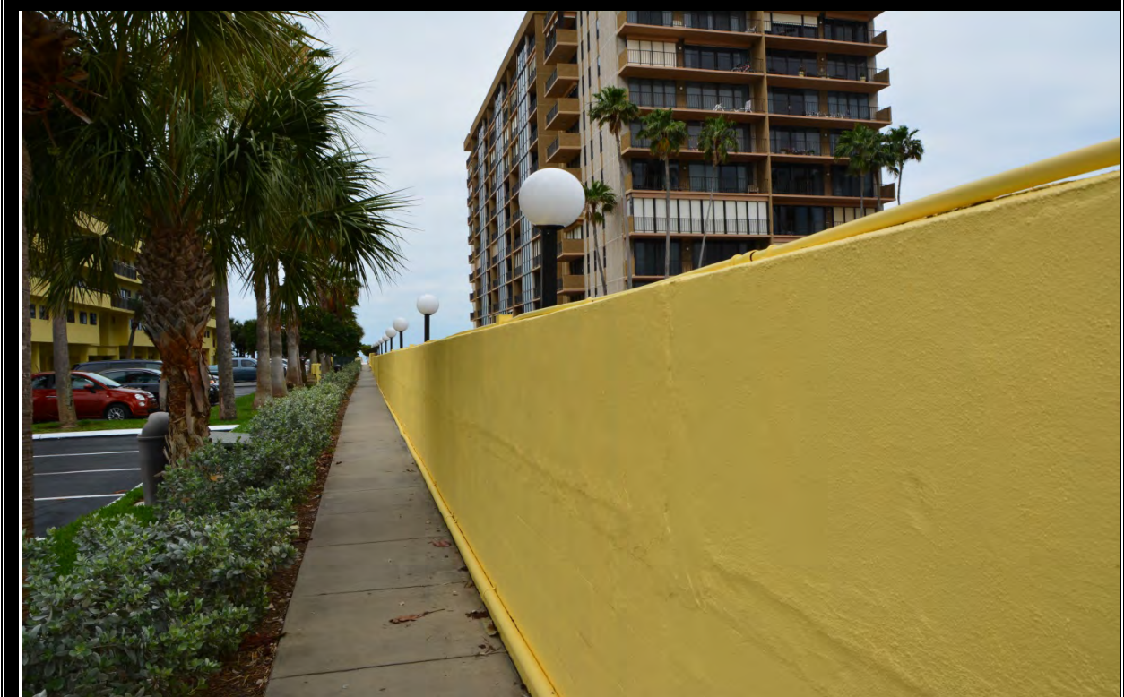
VIEW OF PERIMETER WALL
