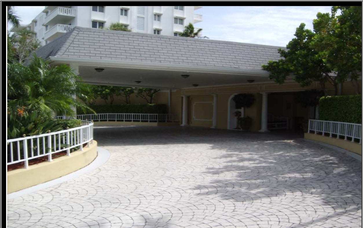
EXTERIOR VIEW OF CLUBHOUSE
