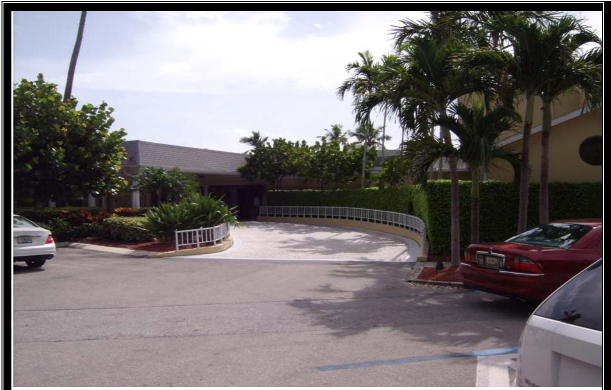
EXTERIOR VIEW OF CLUBHOUSE
