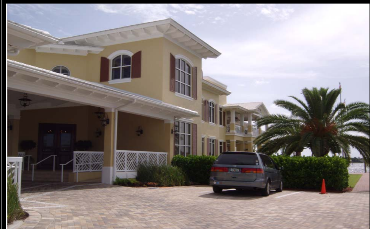
EXTERIOR VIEW OF CLUBHOUSE ADDITION
