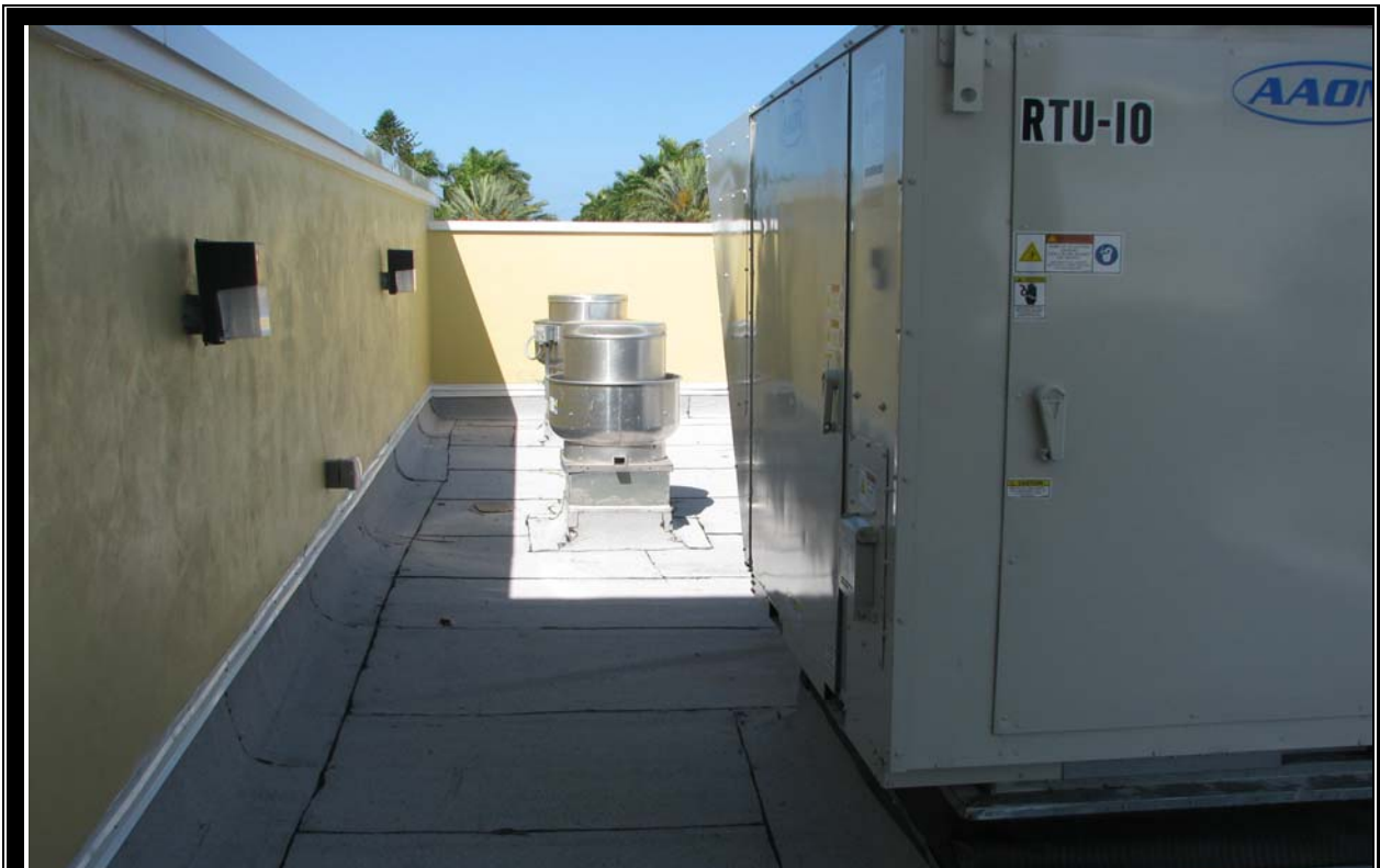
VIEW OF ROOF AND MECHANICAL BUILDING EQUIPMENT
