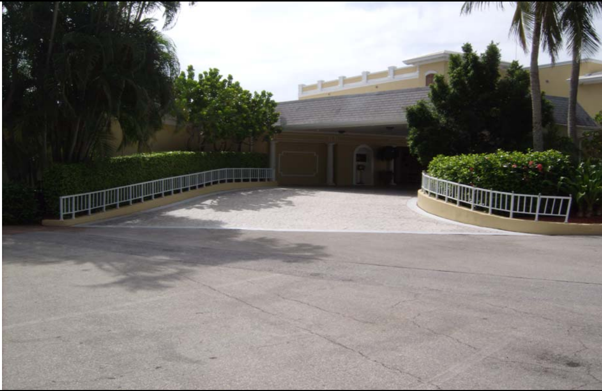
EXTERIOR VIEW OF CLUBHOUSE
