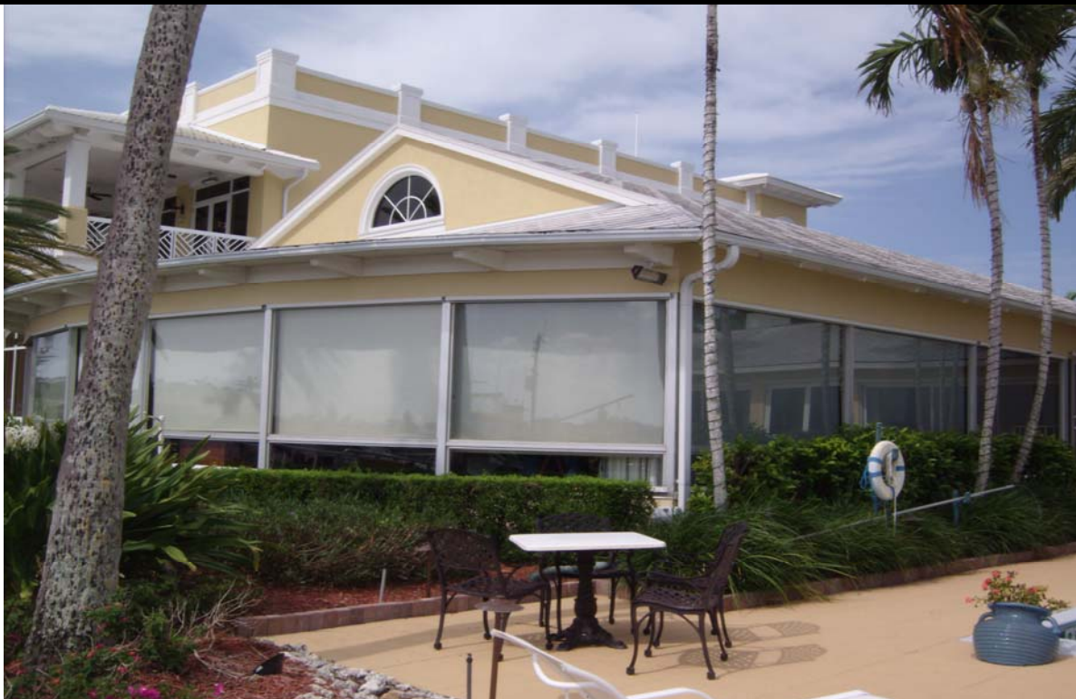
EXTERIOR VIEW OF CLUBHOUSE
