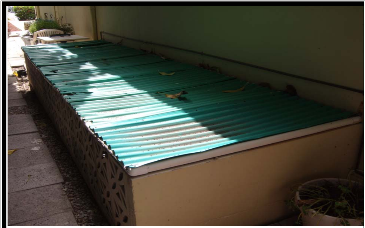
VIEW OF TYPICAL SWIMMING POOL EQUIPMENT
