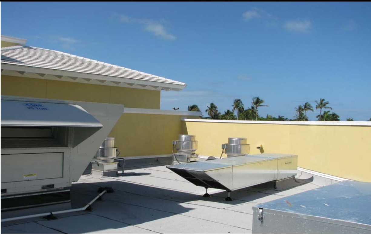
VIEW OF ROOF AND MECHANICAL BUILDING EQUIPMENT
