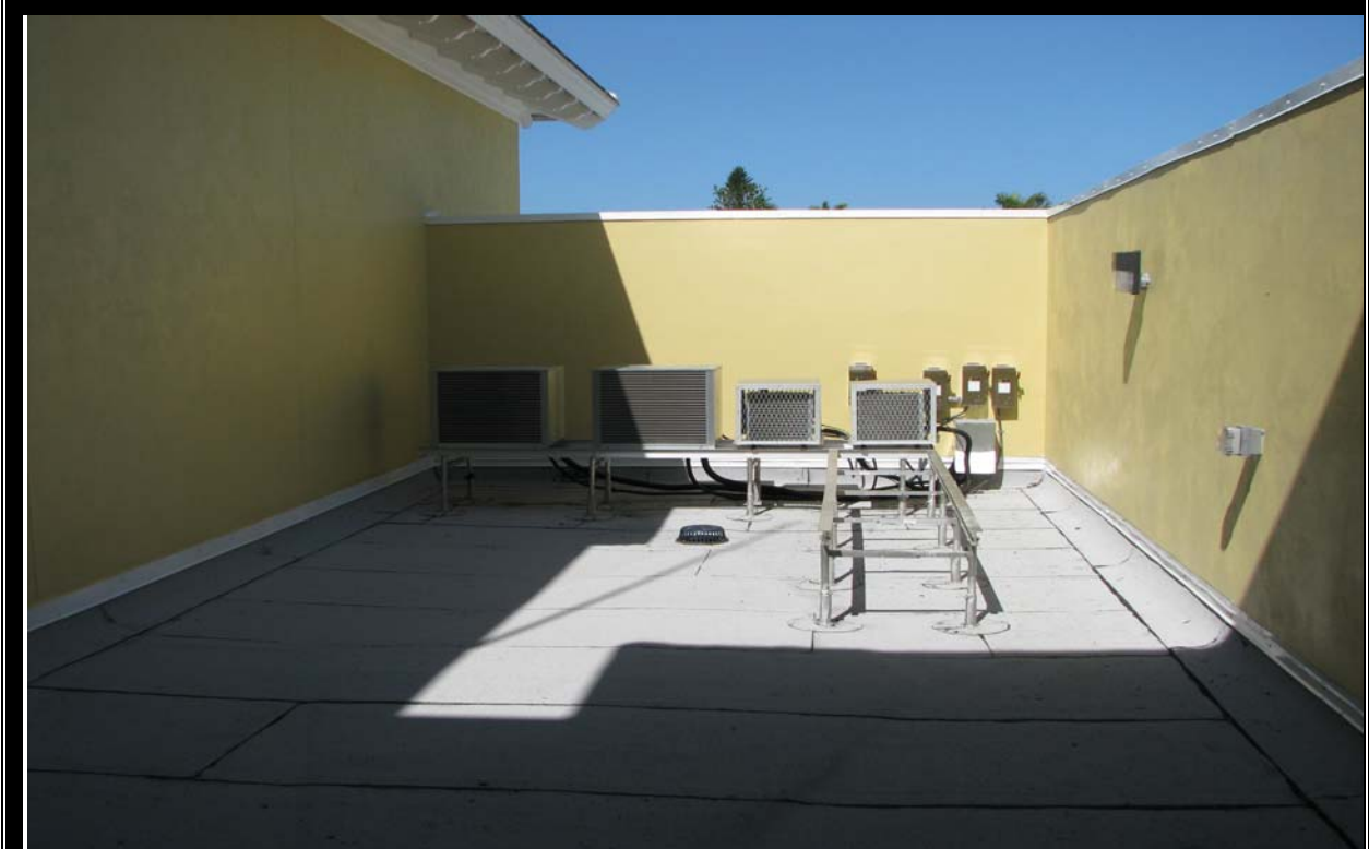
VIEW OF ROOF AND MECHANICAL BUILDING EQUIPMENT
