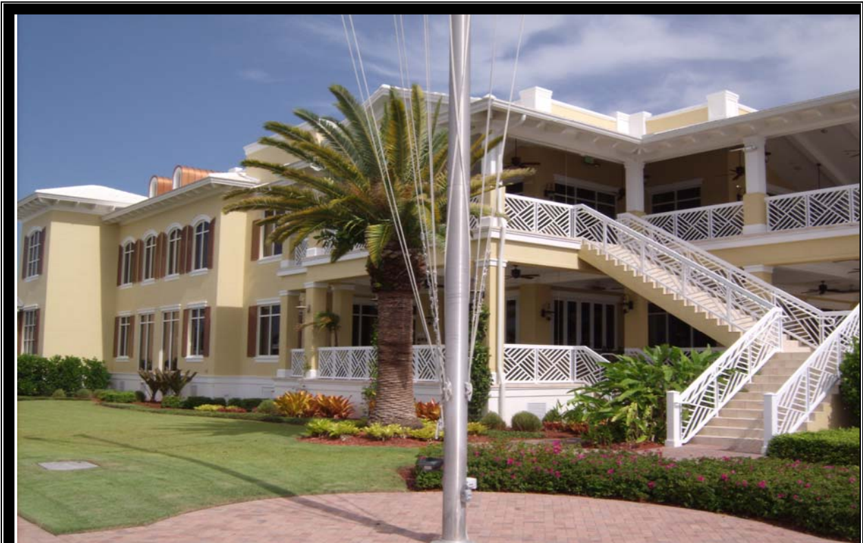
EXTERIOR VIEW OF CLUBHOUSE ADDITION
