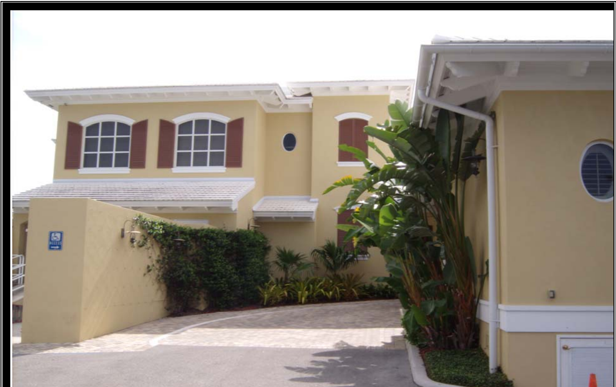
EXTERIOR VIEW OF CLUBHOUSE ADDITION
