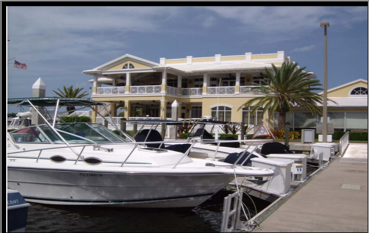
EXTERIOR VIEW OF CLUBHOUSE ADDITION
