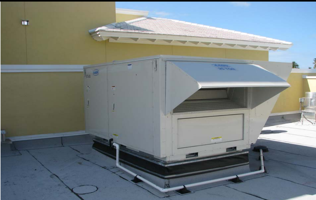
VIEW OF ROOF AND MECHANICAL BUILDING EQUIPMENT
