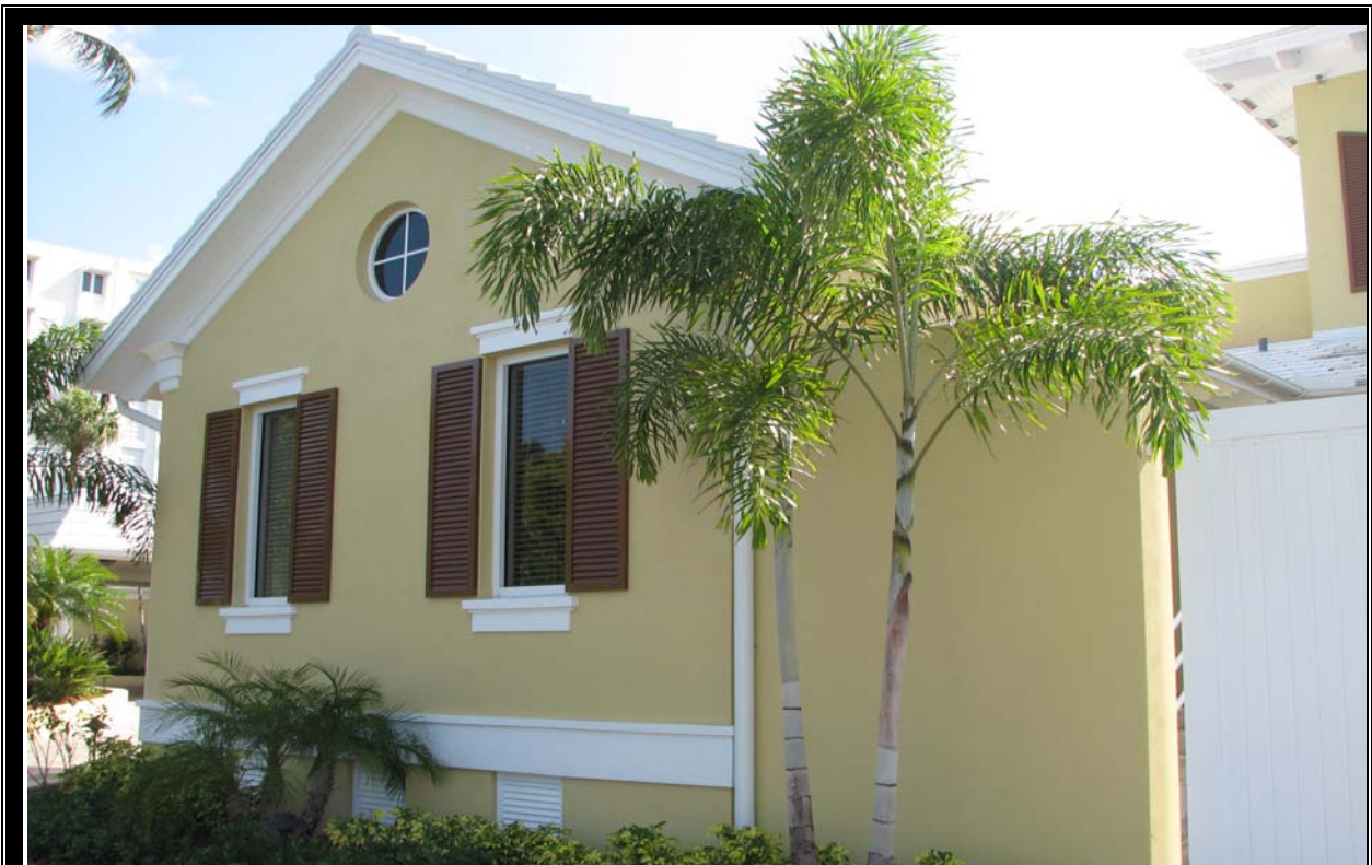
EXTERIOR VIEW OF CLUBHOUSE KITCHEN RENOVATION
