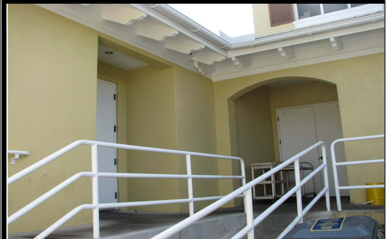
EXTERIOR VIEW OF CLUBHOUSE KITCHEN RENOVATION
