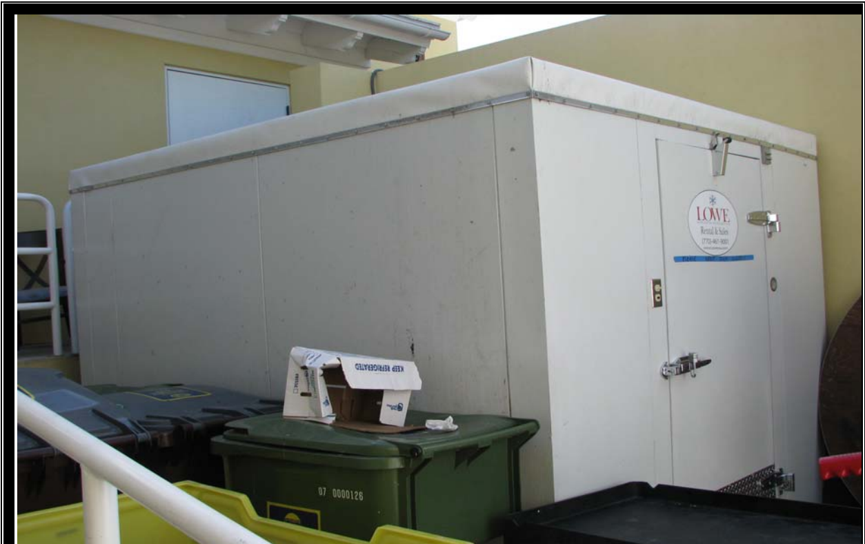
VIEW OF ROOF AND MECHANICAL BUILDING EQUIPMENT
