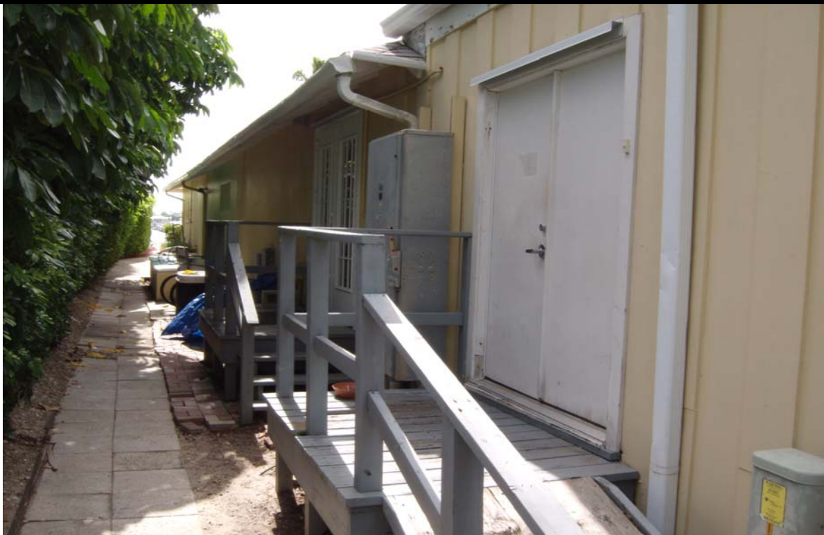
EXTERIOR VIEW OF CLUBHOUSE
