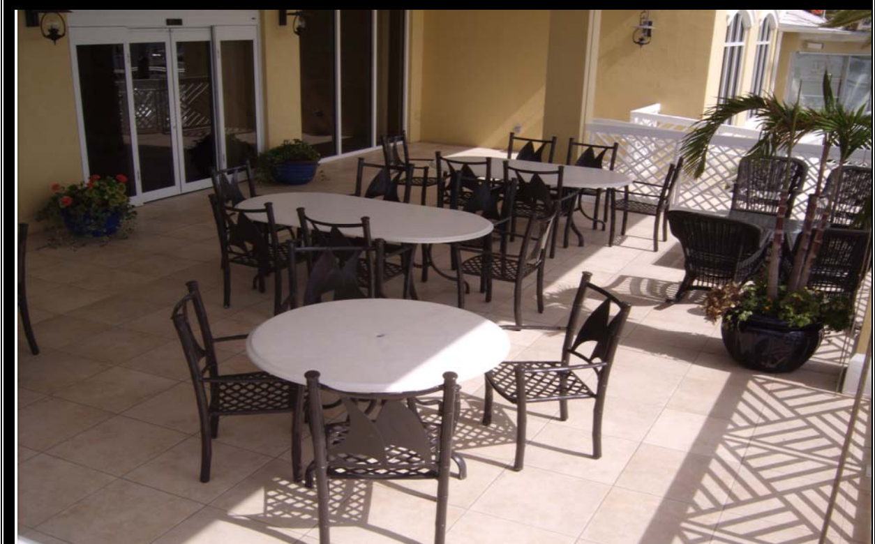
EXTERIOR VIEW OF CLUBHOUSE ADDITION
