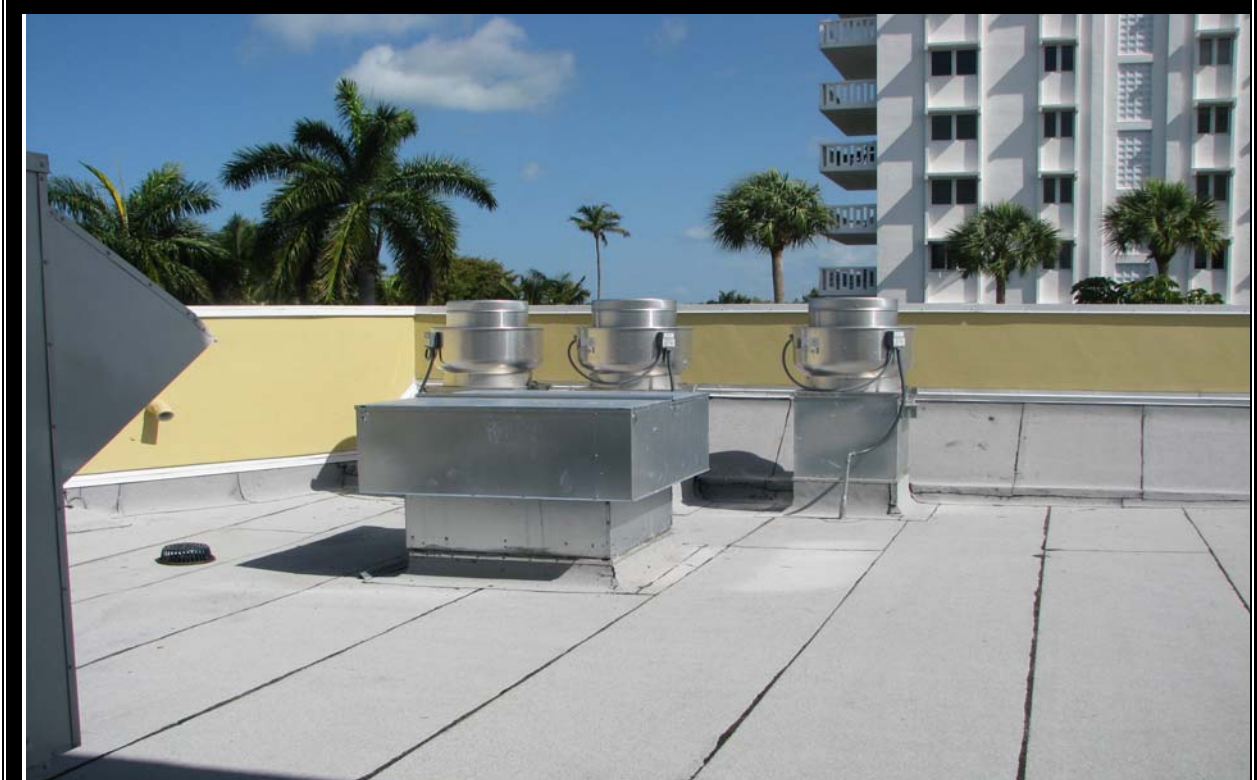
VIEW OF ROOF AND MECHANICAL BUILDING EQUIPMENT
